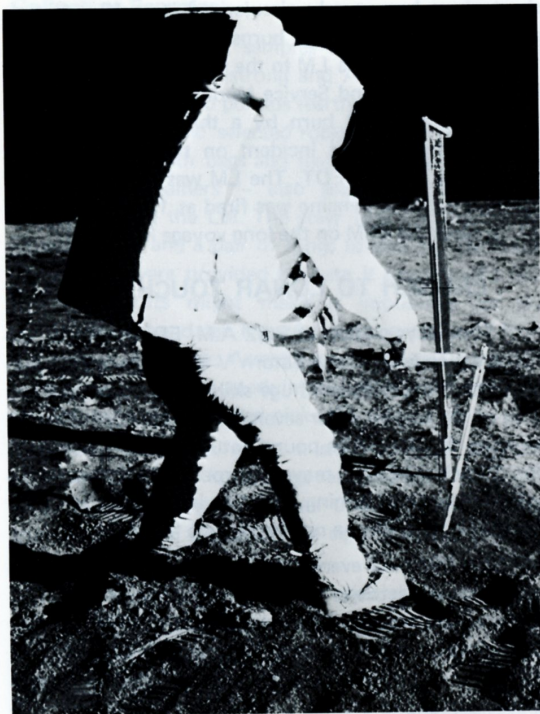
Astronaut Edwin Aldrin is in the process of taking a lunar soil sample. In the background is the solar wind experiment.
