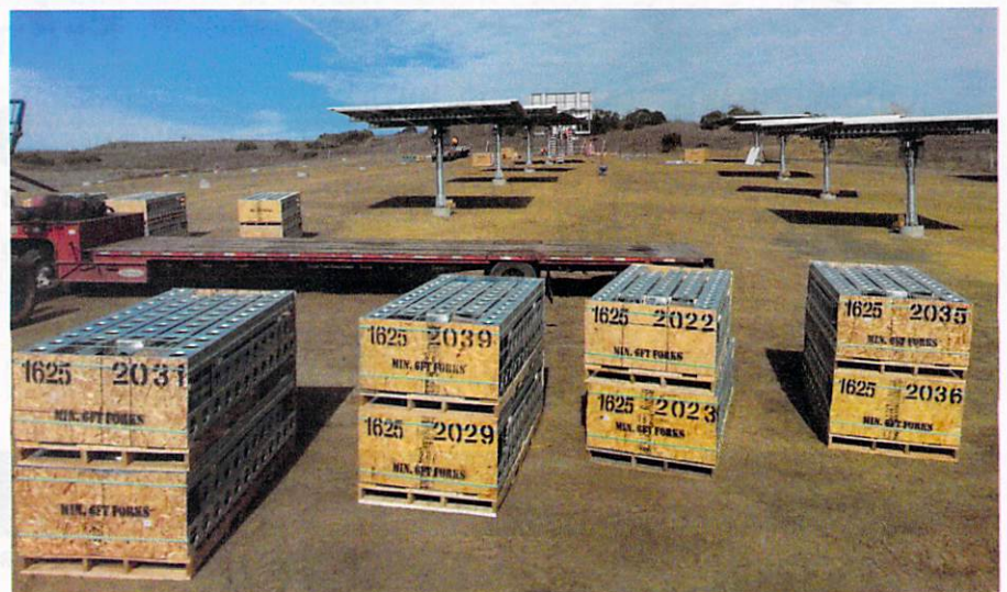
Tracker installation underway at the job site.
