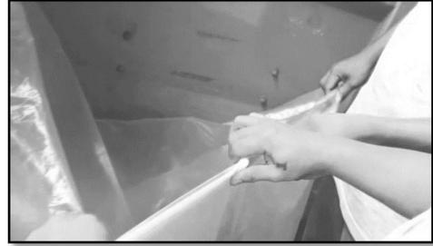
3.3.3. Manually zip a few centimeters enough to initially engage the zipper slider.
