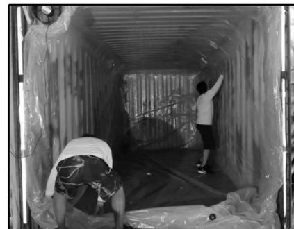
2.1.4. Place cardboards on the TSL floor and along the walls for added protection;
