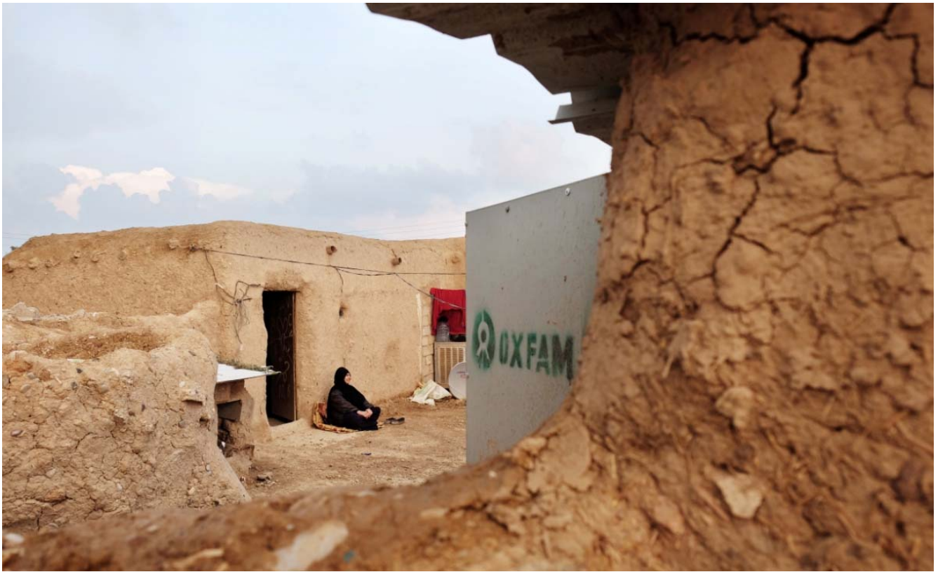
View into a family's home in Hosseini village, central Iraq, where many have begun to rebuild. Photo: Oriol Andres/Oxfam
