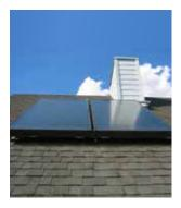
Vitosol 200-F flat plate solar collectors
