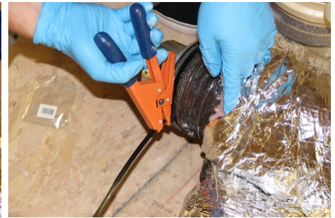
Use tie band and tensioner to secure liner to connection fitting
