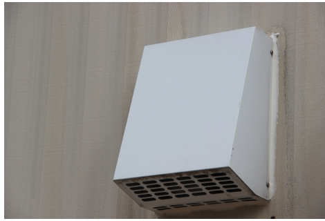
Through the wall exhaust fan sealing.
