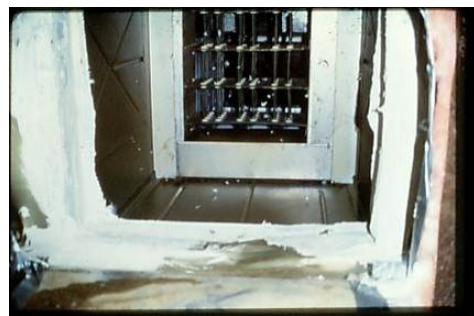
Using mastic and mesh tape, fully seal the furnace to the trunk line. Repair and seal the access holes in duct and belly
