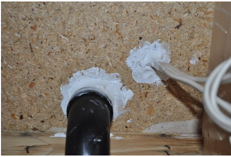
Visually inspect to verify no gaps remain
