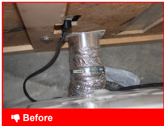
Dryer is vented outside, but with wrong material
