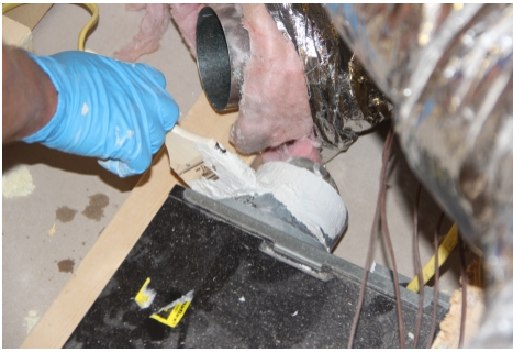
Apply mastic to fan connection
