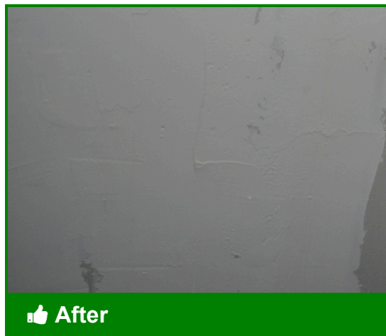
Drywall patch before final sand and prime
