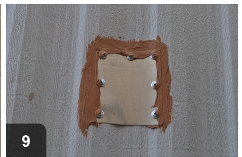
Securely fasten patch in place with screws and apply addition sealant to deter water
