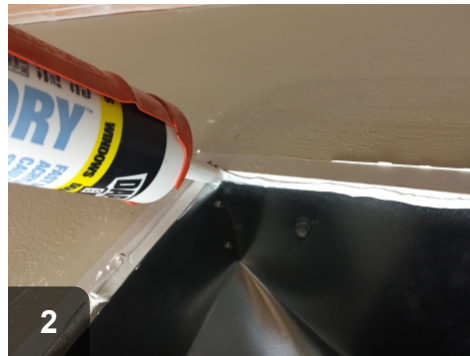
2 Caulk the boot to the gypsum board. Angle the tip forward and force caulk into the joint
