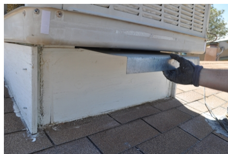
The damper needs to be opened at the beginning of summer
