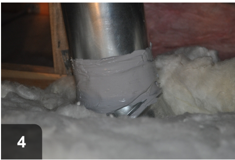
Coat joint with UL-181 mastic, at least 0.08" (2mm) thick
