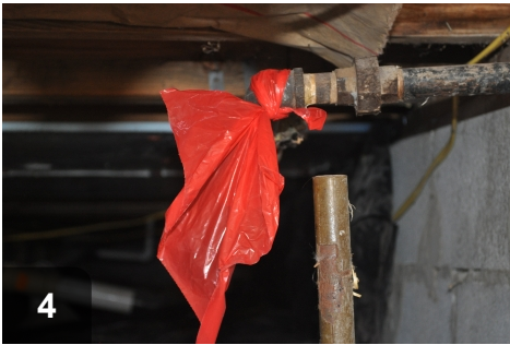
4 Allow testing solution to sit on newly repaired pipe joint for 10min
