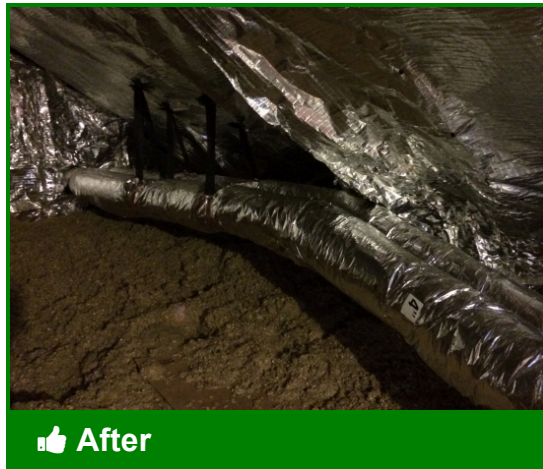
After Fan has been vented with sealed, insulated duct material
