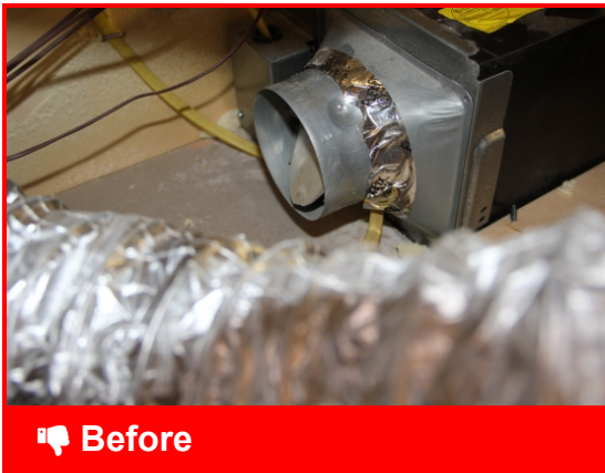
Before Fan duct is disconnected and venting into the attic space.
