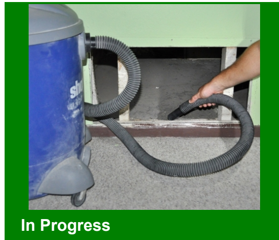
Vacuum out debris and dirt from the return to prepare work area
