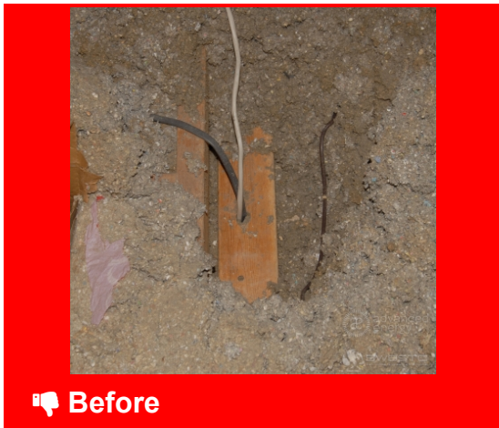
Unsealed penetrations through top plate
