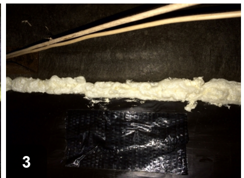
Apply foam or caulking over backer
