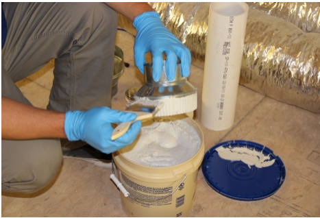
Apply mastic to the connection fitting
