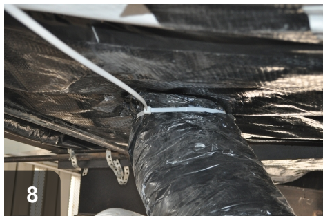
8 Secure insulation and outer casing place with tie band
