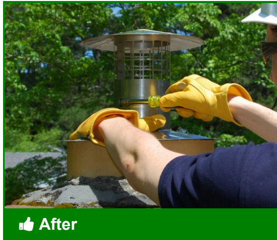
Flue liner with rain cap
