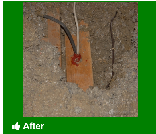
Sealed wiring penetrations through top plate
