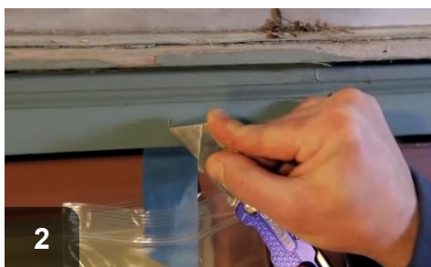
2 Place catchment bag under sample site to catch any debris. Cut sample site at an angle to expose all older paint layers
