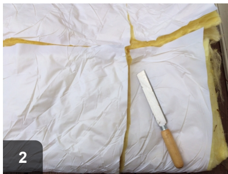
2 Wrap blanket around tank and mark it where it overlaps. Add two or three inches and cut off using a straightedge and raz
