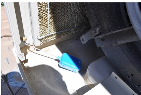
The float, attached to the water valve, shows no signs of cracking
