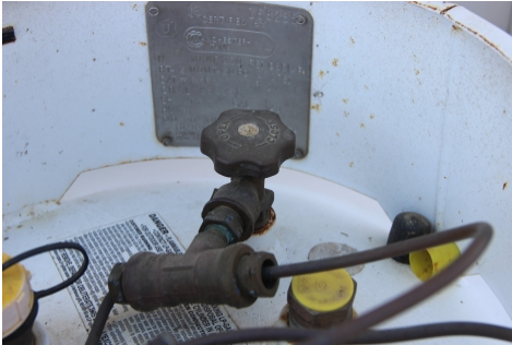
Propane - Ensure gas valve is open at the tank and there is fuel in the tank
