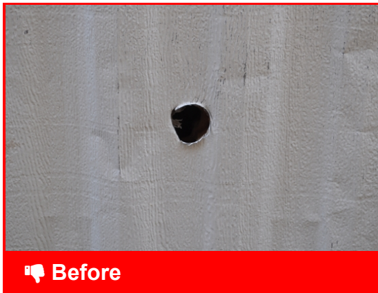
Hole in exterior wall of manufactured home aluminum siding
