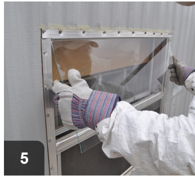
Install new glass, ensuring 1/8" gap from frame on all sides
