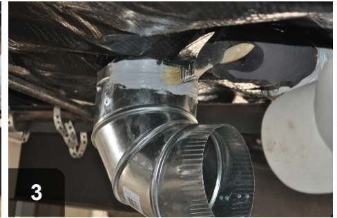
3 Apply mastic at metal-to-metal connection
