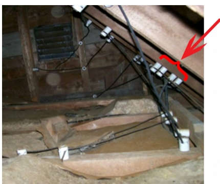
Recognize if knob and tube wiring is present and take special precautions
