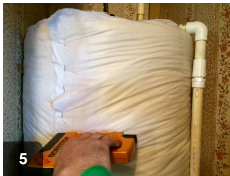
5 Staple the flap to the blanket with outward clinching staples or use long zip ties to secure the blanket in place
