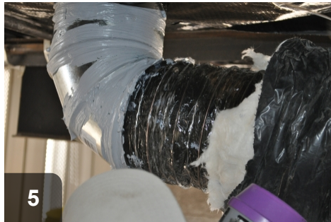
5 Slide inner liner onto flange with sealant
