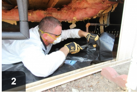
2 Measure, cut, and spread vapor barrier material after removing debris over 1/2" in size. Notch around obstructions
