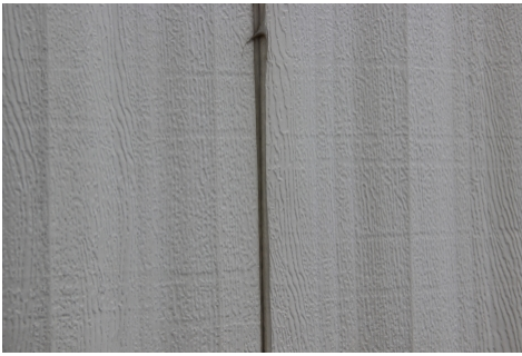
Seams on aluminum siding must be tight.
