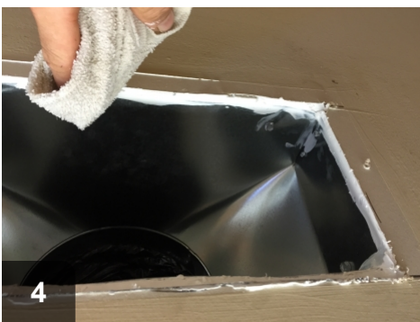
4 Wipe away excess caulk (use water on siliconized acrylic, alcohol on silicone, and solvent on polyurethane caulk)
