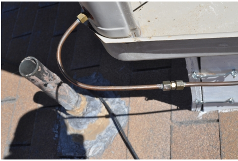
Water line is in tact and not leaking
