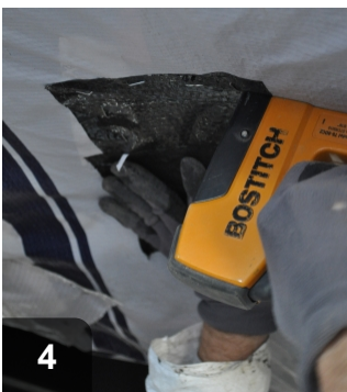
Stitch staple patch to securely fasten physical barrier
