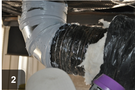
2 Slide inner liner onto flange with sealant
