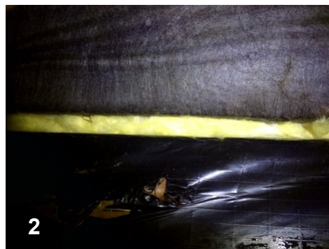
Stuff wide gaps in the marriage line with fiberglass insulation or foam backer rod before applying sealant
