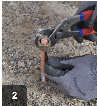
2 Attach grounding wire to grounding rod with acorn coupler
