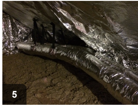
Wrap duct with R-8 insulation. Seal seams in insulation vapor barrier with UL-181 listed foil or Mylar tape
