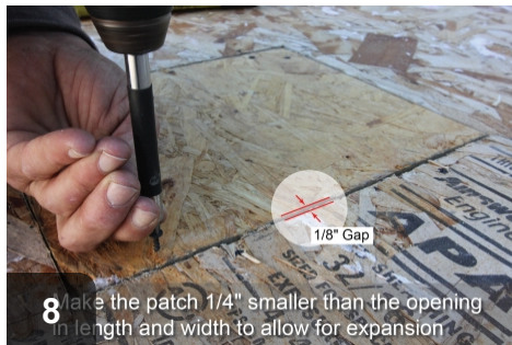
8 Fasten with 2" deck screws
