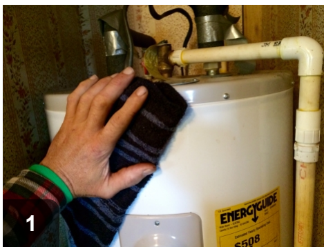
1 Clean the entire outside of the water heater
