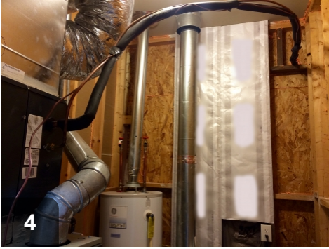
Complete installation by adding supports and fasteners as required for stability and durability
