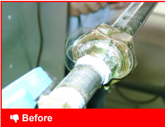
Fuel lines should be inspected for leakage
