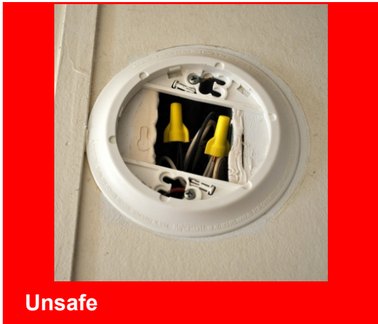
Hard-wired smoke alarm mount with alarm missing
