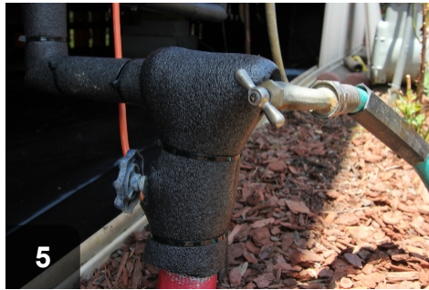
Cover all exposed portions of the water supply lines with insulation
