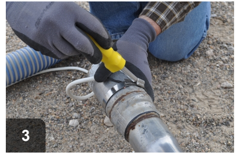
3 Attach grounding wire to metal fill tube with metal coupler
