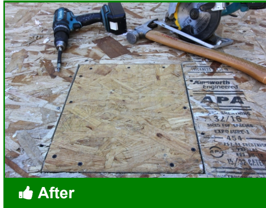
Completed floor repair
