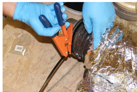
Use tie band and tensioner to secure liner to connection fitting
