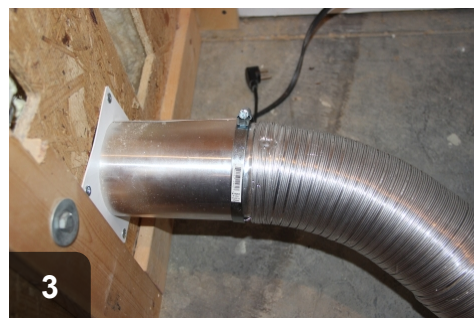
Attach approved vent material to termination vent. Termination vent may need to be trimmed.
