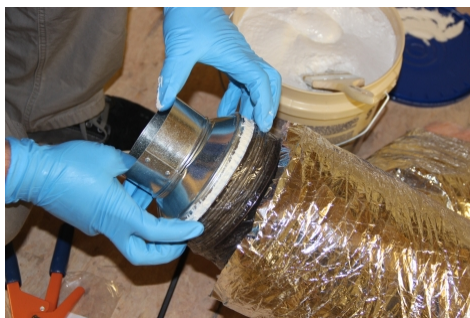
Snug duct liner onto connection fitting
