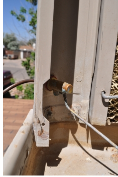
Water valve has signs of deposits, but isn't leaking
