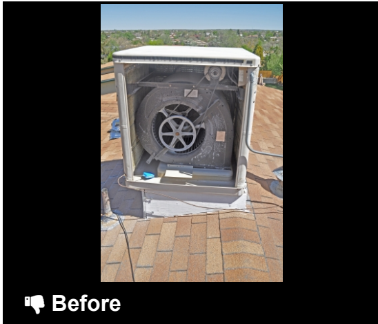
Assess wear and tear on various parts of evaporative cooler
