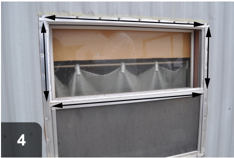
Run sealant bead around entire sash to seal glass from the interior
