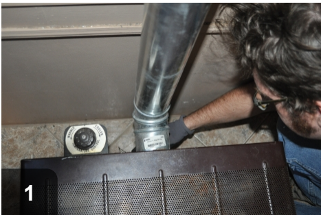
Inspect appliance for evidence of damage or unsafe operation before testing
