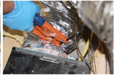
Snug insulation to fan housing and strap into place
