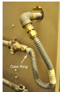
Inspect flex lines for damage, and check date on ring for pre-1973 hardware
