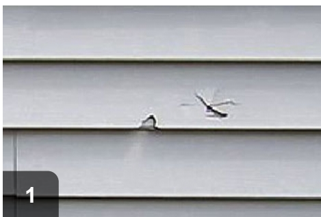
Replace damaged siding
