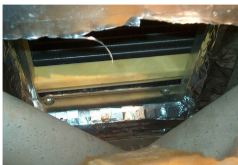
Create an opening large enough to completely seal the plenum to the trunk line
