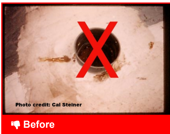
Roof leak, missing cap on vent
