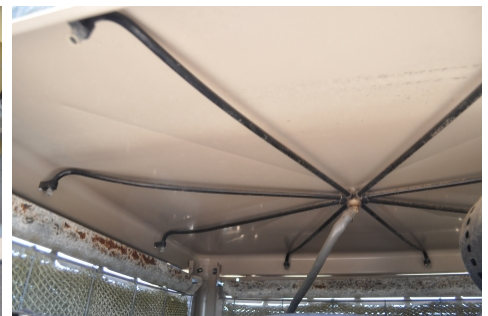
Check spider, which distributes water to pads, for cracks and leaks
