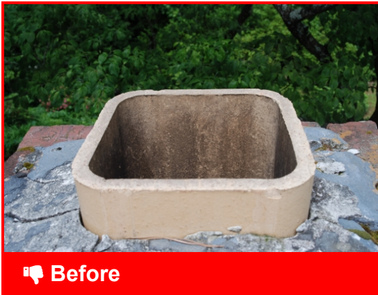
Unlined masonry chimney
