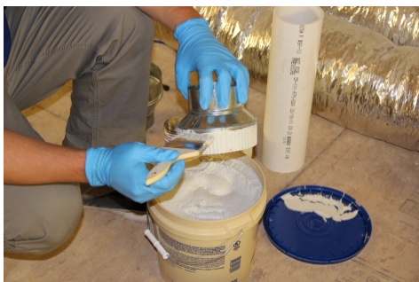
Apply mastic to the connection fitting
