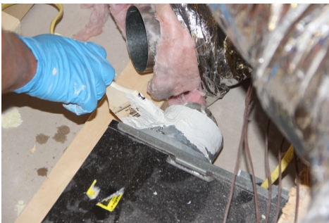
Apply mastic to fan connection
