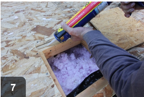
7 Apply subfloor adhesive to nailers
