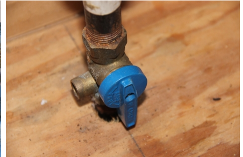
Ensure gas valve is open at the appliance
