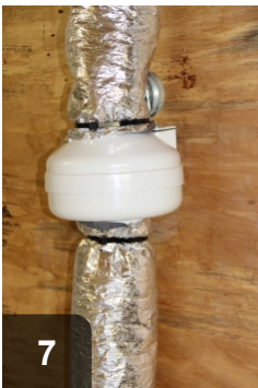
7 For vent runs >35 feet, a booster fan is required.
