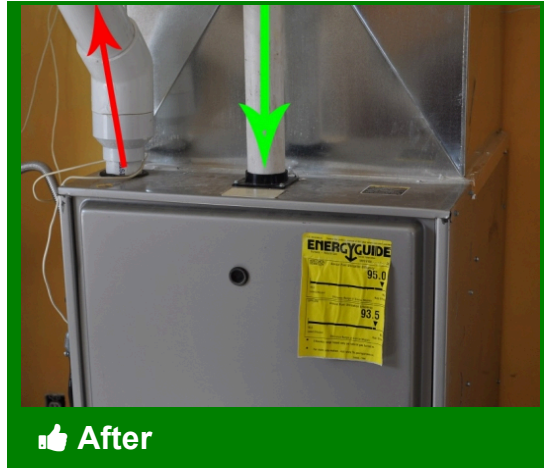
Sealed-combustion, direct-vent appliances should replace unsafe appliances
