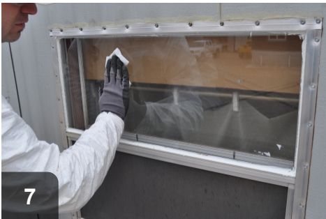
Clean glass to ensure than no out of place adhesive or glazing remains to bake onto glass
