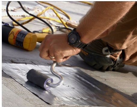
Forcefully roll the patch into place, starting from the center and working toward the edge.
