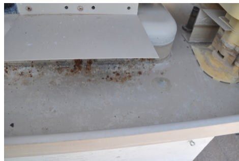
Pan has calcium deposits as well but still holds water
