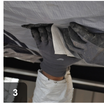
Use adhesive patch to air seal
