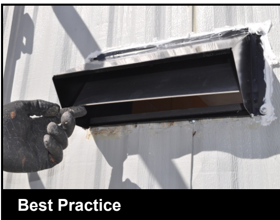
Kitchen exhaust termination fitting should include a backdraft damper
