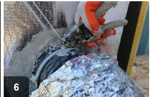
6 Secure with properly tensioned zip tie.
