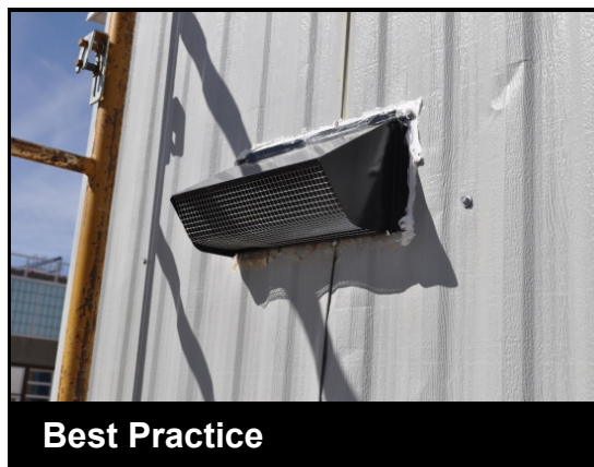
A screen can also help to discourage vermin infiltration
