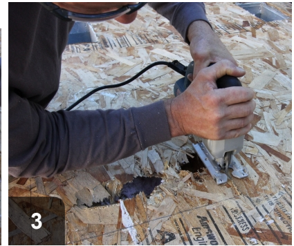
3 Cut out damaged area even with the inside edges of the floor joists
