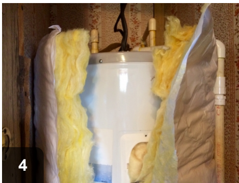
4 Pull insulation blanket around the tank
