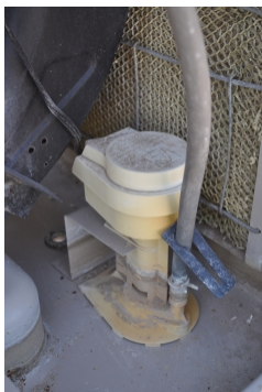
Pump needs to be cleaned of calcium deposits
