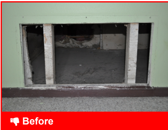
Dirty, unsealed return platform needs to be cleaned out before sealing
