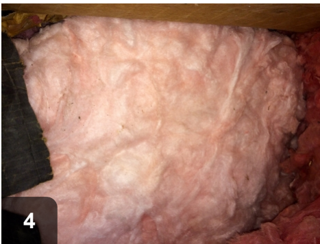
Replace or reinstall fiberglass belly insulation
