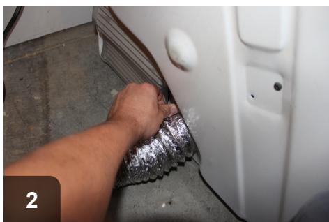
Disconnect existing vent pipe from dryer.
