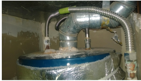
Inspect for missing draft diverter
