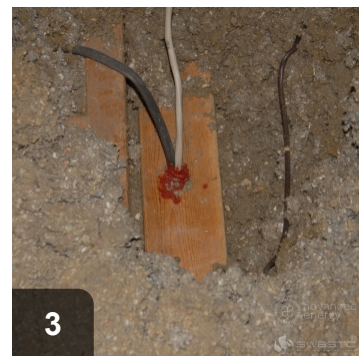
Ensure that all accessible gaps, holes, and penetrations are filled
