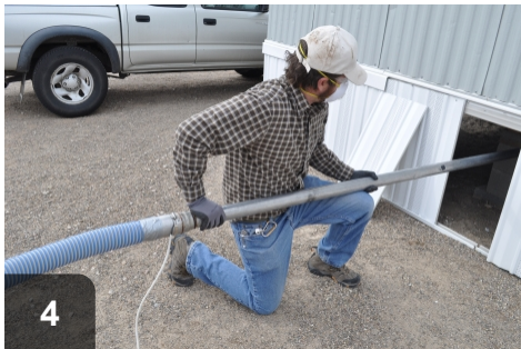
4 Proceed with blowing insulation without fear of static shock
