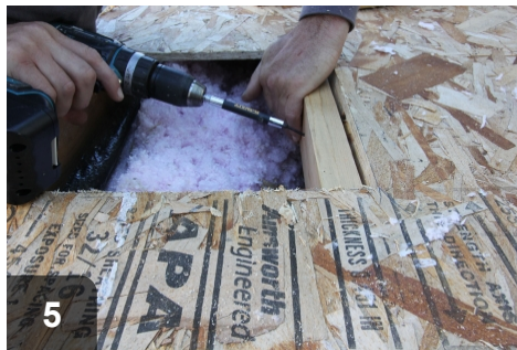
5 Install nailers flat against the joists. Finish by toenailing or screwing 2X4s between the joists
