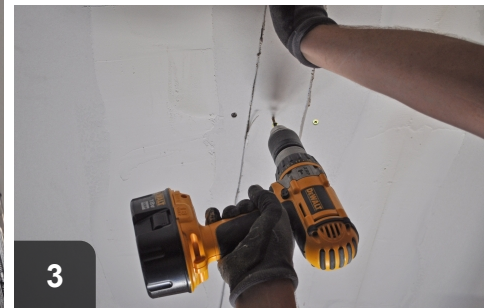
Cut drywall and fasten in place
