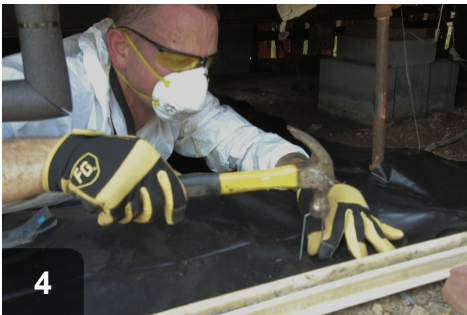
4 Secure vapor barrier to ground with corrosion-resistant landscape staples, or weigh it down with ballast
