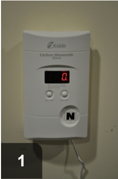
1 Mount alarm to wall close to bedrooms
