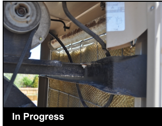
Pads have deposits and are shrunken from age. Replace
