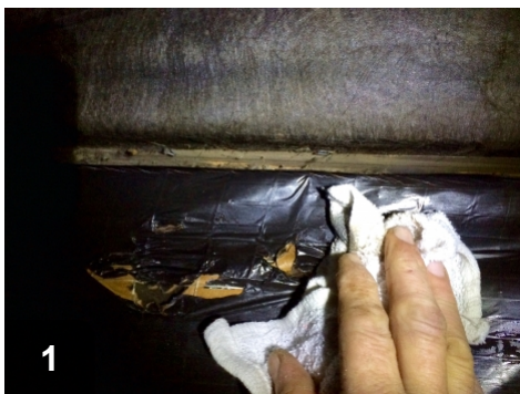
Clean belly wrap before air sealing
