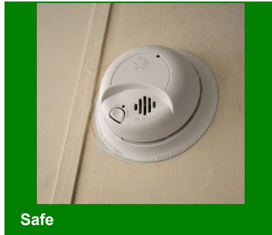
Hard-wired smoke alarm mount with alarm replaced
