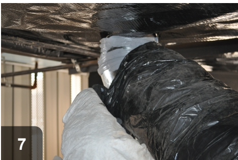
7 Extend insulation and exterior casing up over elbow until they reach belly
