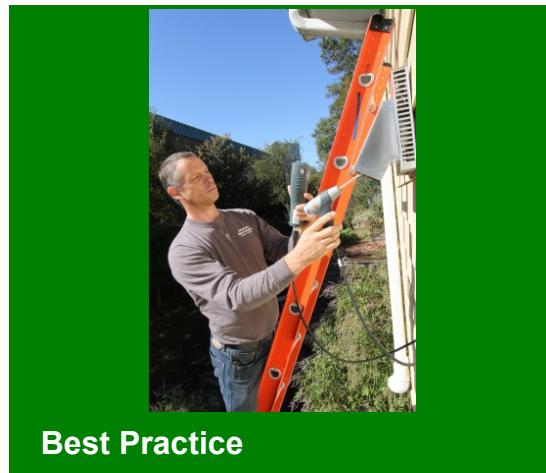
Check carbon monoxide levels in the appliance vent
