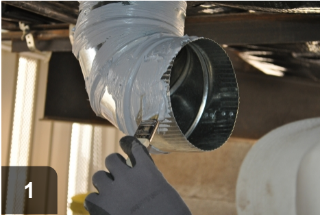
1 Apply mastic to flange
