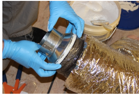
Snug duct liner onto connection fitting
