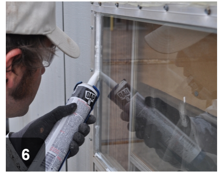
Apply glazing or install replacement stops to seal window from exterior
