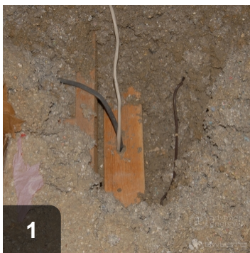
Locate and expose penetrations to prepare for sealant
