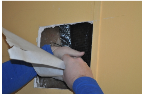
Patch holes in air and/or vapor barriers as well
