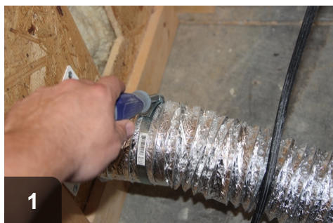
Disconnect existing vent pipe from termination. If hose clamp is installed, save for reuse.
