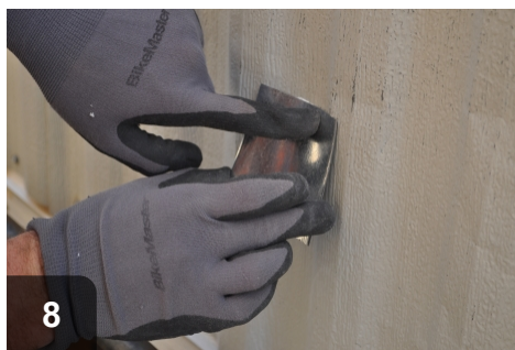
Flex patch to contour to wall
