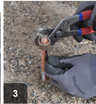
3 Attach grounding wire to rod with coupler
