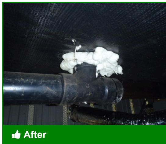
Properly sealed penetration through manufactured home bottom board
