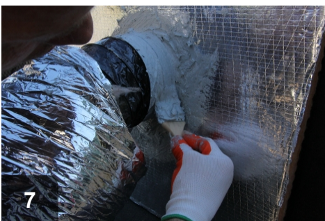
7 Coat seam with mastic
