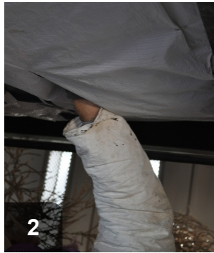
Holes in belly air barriers allow vermin access to insulation and ducting
