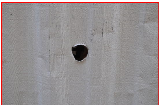
Hole in exterior wall of manufactured home aluminum siding
