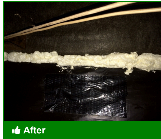
Completed air sealing at marriage line
