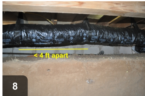
8 Duct runs outside of conditioned space must be properly supported.
