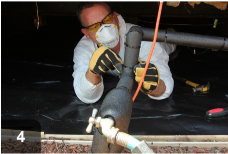
Fasten insulation to water lines with zip ties
