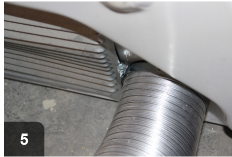
5 Connect vent pipe to dryer.
