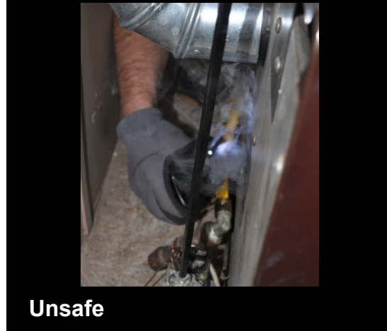
Spillage should not exceed 2 minutes, if present
