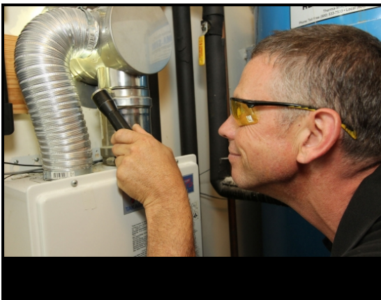
Inspect direct vents for proper connections, rust, corrosion, and clearances
