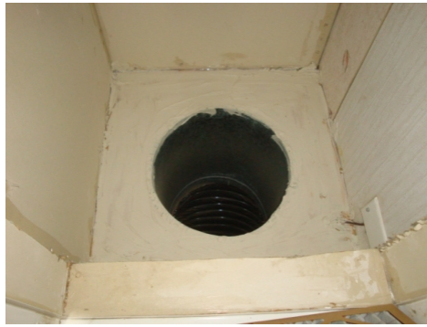
Apply mastic to inside seams of plenum
