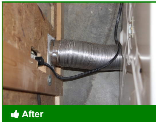
Dryer is vented outdoors, with correct material. Run is as short and straight as possible ensuring maximum flow.
