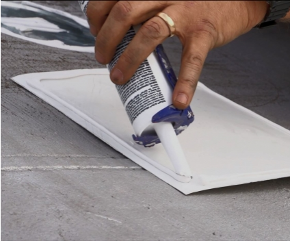
Apply sealant to the underside of the sheet metal patch.
