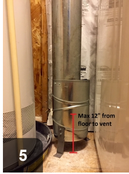
Terminate low vent within 12" of the floor. This one is fastened to a section of larger diameter duct for stability
