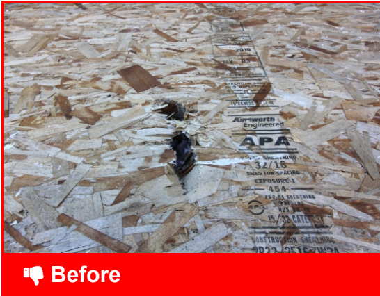
Remove floor coverings from damaged area
