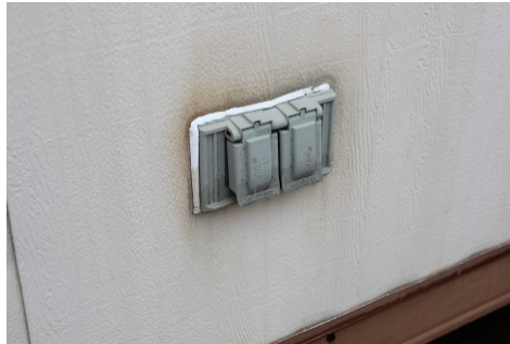
Exterior electrical outlet sealing.
