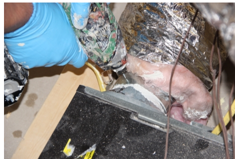
Using mechanical fasteners, secure connection fitting to fan connection
