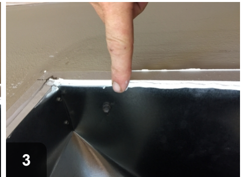
3 Wipe the caulk into the joint and smooth it as you go
