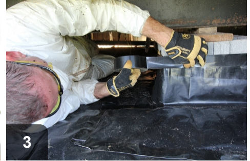
3 Wrap piers and columns at least six inches high. Use additional material to cover any gaps and holes in vapor barrier
