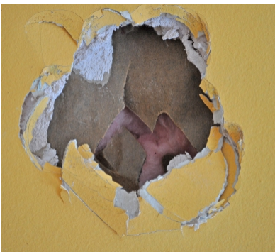
Patch holes in air and/or vapor barriers as well
