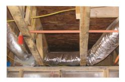
"The Lane housing units have wood construction, which made the labor savings with the BlazeMaster CPVC system even greater than it would have been using a steel frame," said Crosswy. "The inconsistencies of a wood frame necessitate the use of CPVC. We wouldn't attempt wood construction on a tight schedule with a metallic fire sprinkler system. It just doesn't make sense."
