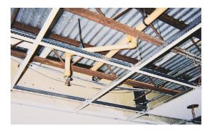
In fact, in one summer, Worsham installed approximately 1,600 sprinkler heads, consisting of 800 heads to NFPA 13 standards in one residence and 800 heads to NFPA 13R standards in two others. According to Chris Lyons, job foreman, "No way could we have met this schedule without the CPVC Piping System."
