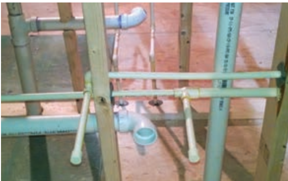
FlowGuard Gold CPVC in Trunk and Branch Configuration
