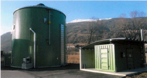
Anaerobic sludge stabilization and energy generation LIPP KomBio Reactor with CHP and condenser unit
