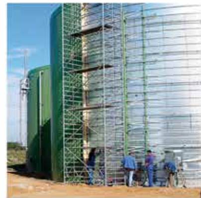
LIPP Universal digester during construction
