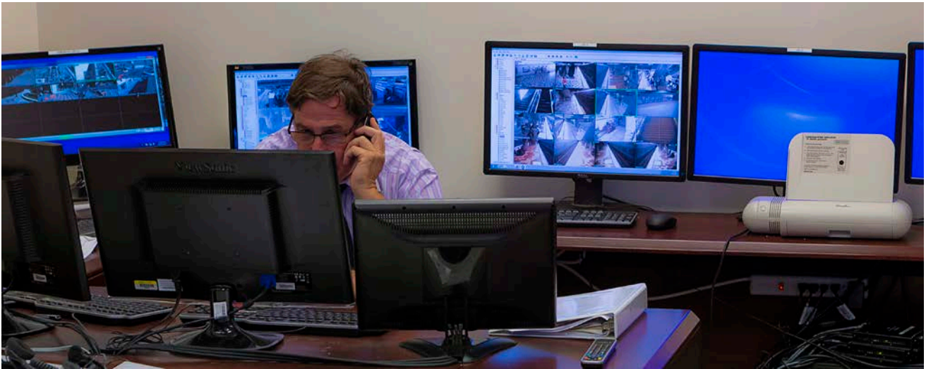
The main Hiperwall video wall room at LA Metro has a station in the back corner, shown above, where the Hiperwall is controlled.
