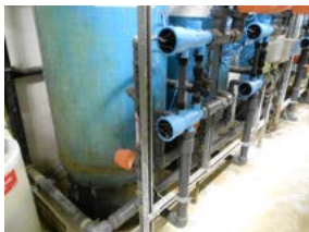
CAD Plant prior to commencement of work
