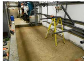
Bund cleared and ready for re-coating
