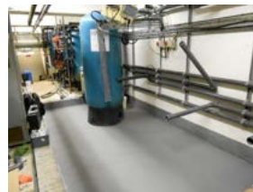
Start of rebuilding
