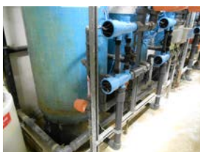
CAD Plant prior to commencement of work
