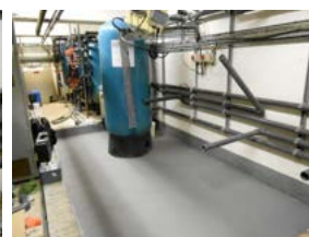
Start of rebuilding
