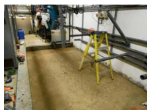
Bund cleared and ready for re-coating
