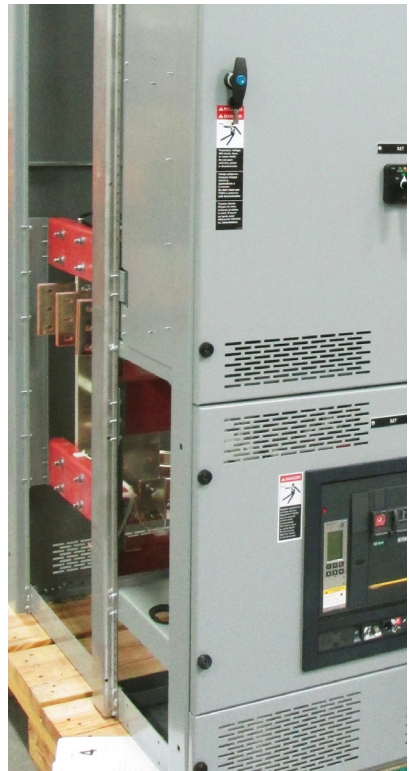
Figure 4: UL 891 Distribution Equipment - If this were UL 1558 equipment, panels would separate the front of the enclosure from the rear, and side panels would enclose the left side.
