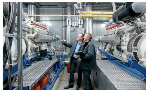
and 3.5 MW of thermal output supplies all of the electricity needed to power lighting, cold store doors, offices and information technology equipment. Surplus power is fed into the public utility grid. The heat that is recovered from Nordfrost's CHP modules is used for heating in the winter, and is also used in combination with absorption chillers for the warehouse's refrigerated storage areas.
