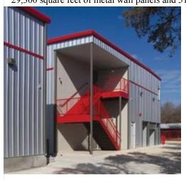
,000 square feet of standing seam roofing. ARCHCON Architecture designed the solar shading, tube steel stairs and railings, which were all custom fabricated by Lobo Steel, Adkins, Texas.
