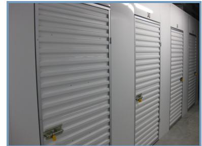
**Roll up doors** are attached to a barrel and coil around it when raised. Roll up doors typically come in wider sizes than swing doors. Swing doors and roll up doors can be interspersed, depending on the size of your units. It is quite common to use swing doors on 5'-0" wide units or smaller and roll up doors on units larger than 5'-0" wide. Renters tend to like having the maximum size doors on units to make it easier to get in and out of their unit.
