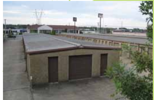
Roll-up doors were not uniform in color, adding to the tired look of the pre-renovated facility.
