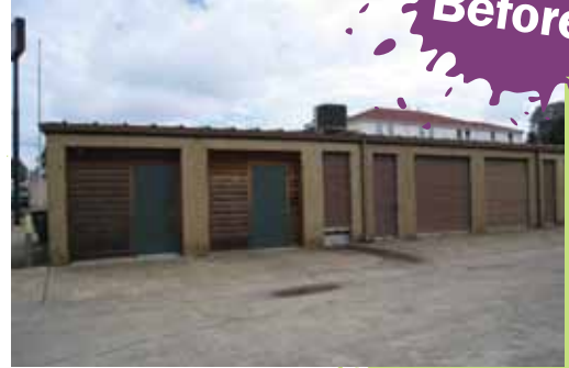
Worn roll-up doors were faded and poorly operational.
