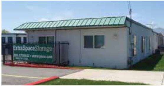
Extra Space Storage in West Jordan, Utah, just prior to renovation.
