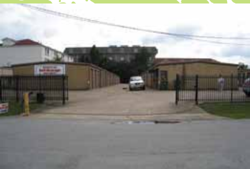
A view of the facility entrance prior to renovation.
