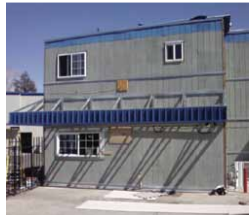
A-American Storage during renovation, with the horizontal wall girts ready for new siding to be attached.
