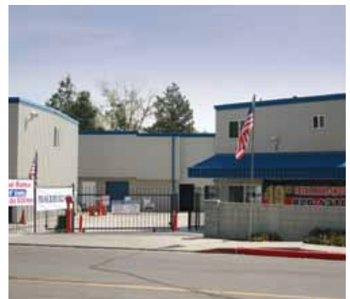
The completed A-American project.
