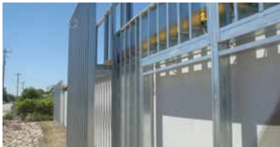
The Extra Space exterior, framed and ready for its new store-front look.
