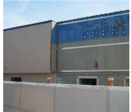
A-American Storage with the old roof and wall trims removed.
