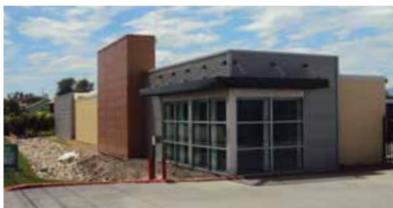
The office renovation, with new windows, siding, canopies, walk paths and exterior paint.
