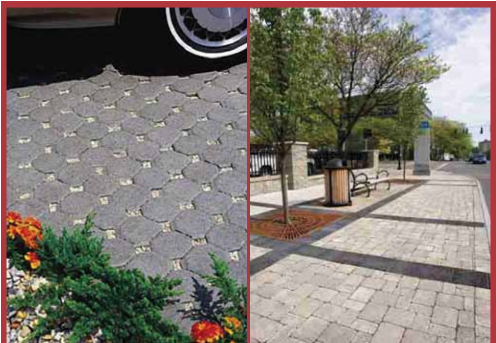
Permeable CMU site pavers allow stormwater to penetrate into the soil, thus avoiding unwanted run off, reducing pollution, and reducing the heat island effect.
