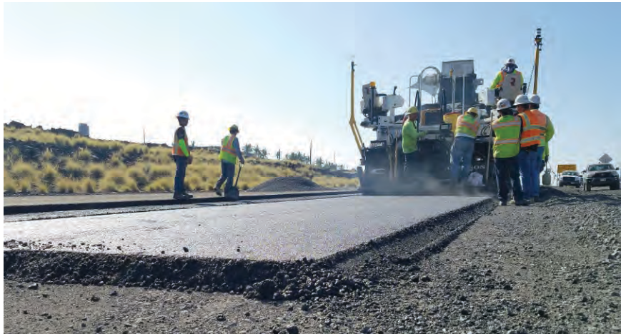
▲ Typically, paving removes 70-80% of low spot deflection with each pass so you may be able to smooth a low spot relatively well before the finishing layer, but compaction will always cause some form of longitudinal waves. An uncompacted design compensated for that.
