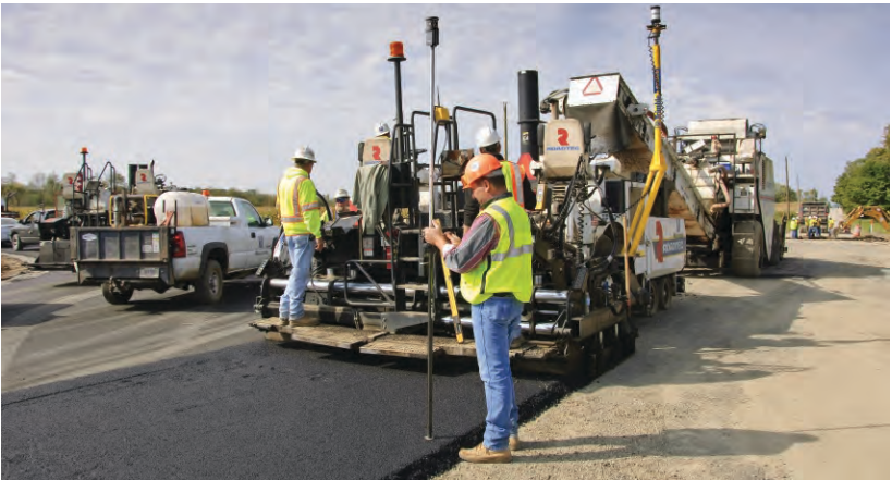
▲ The result of 3D paving with an uncompacted design is a smoother surface with less effort and less material as it eliminates the need for a leveling course.
