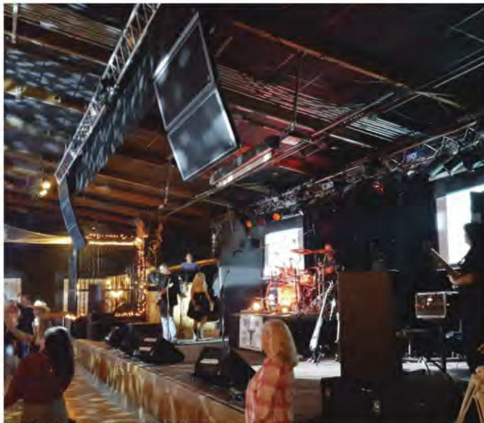
The Saddle Rack's main P.A. features six Tectonic PL-12 Plate flat panel speakers.
