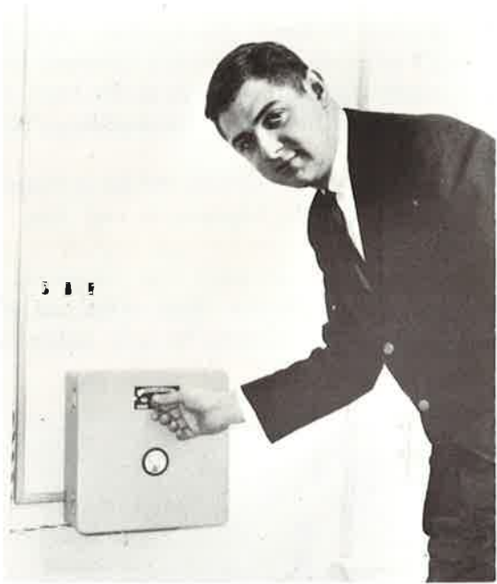
Greg Doyle, General Manager of Bureau, next to panel housing junction of two circuits of alarm.
