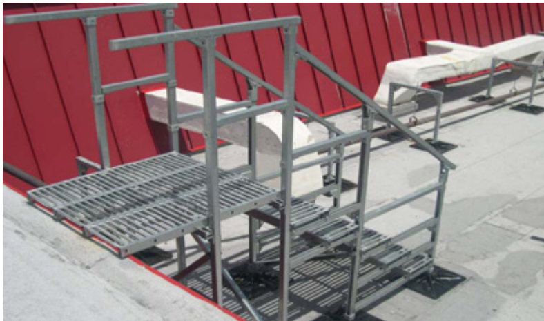
Access stairs with handrails
