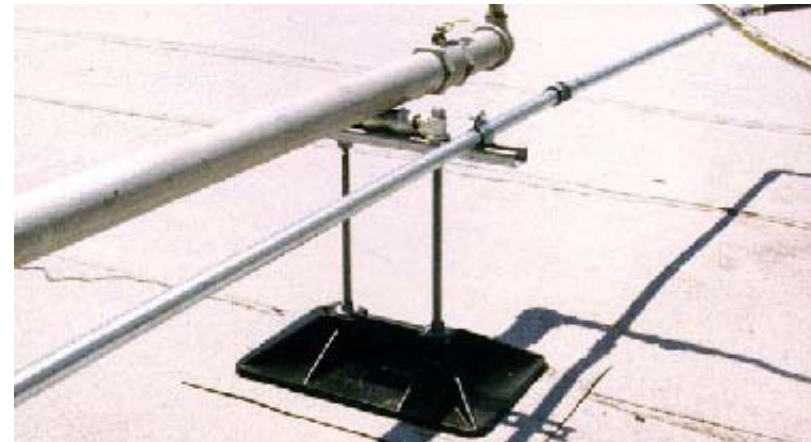
Height adjustable support with channel and roller supporting conduit
