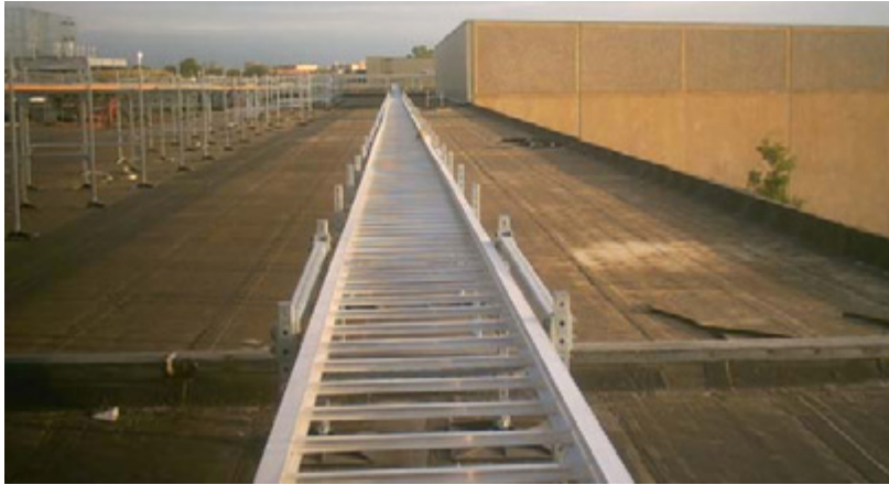
Over 3,000 lineal feet of cable tray ranging from 12" to 36" wide and 36" above finished roof
