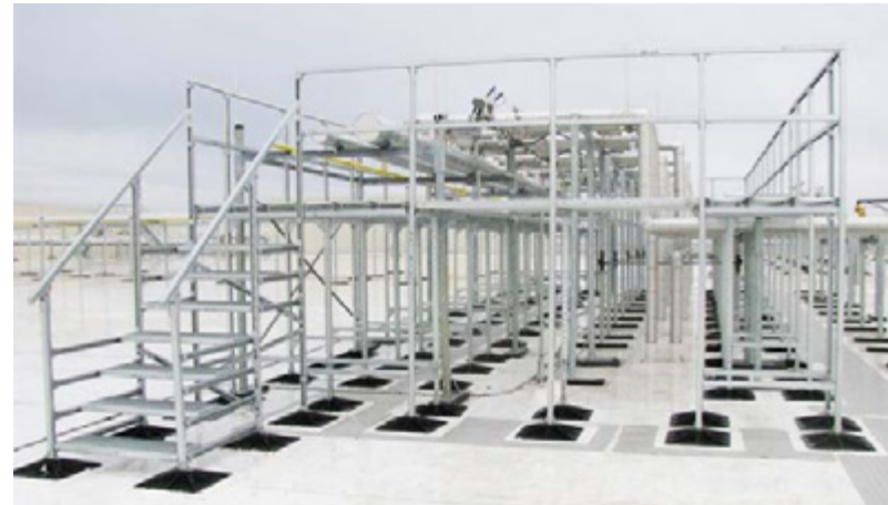
Access platform with stairs
