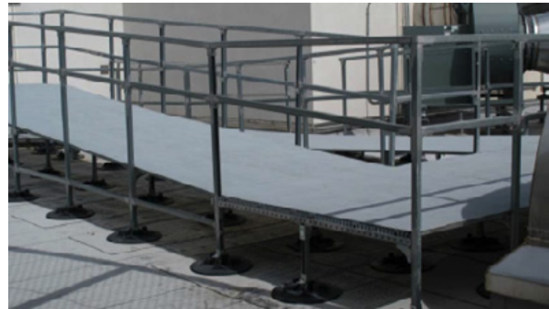
Ramp system with stair access
