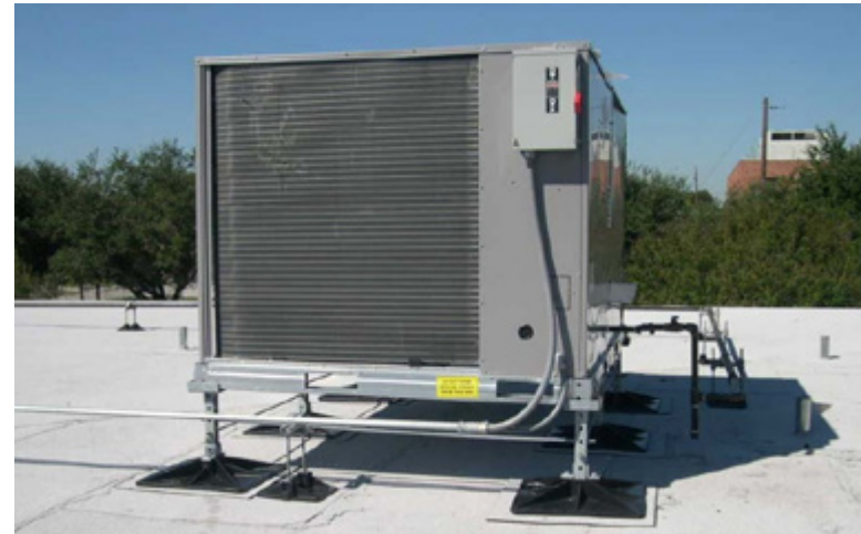
HVAC with corner and center supports and with electrical and gas supports
