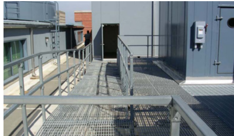
Ramp and walkway system with handrails
