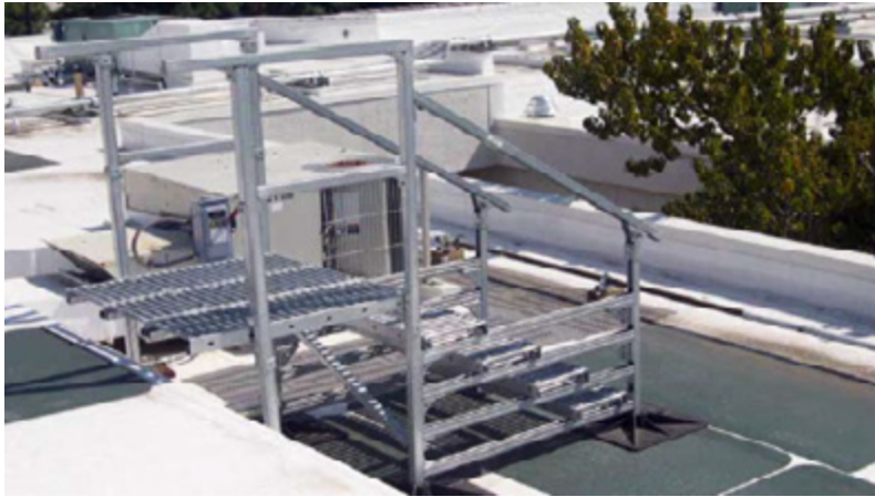
Roof-to-roof access stairs with handrails
