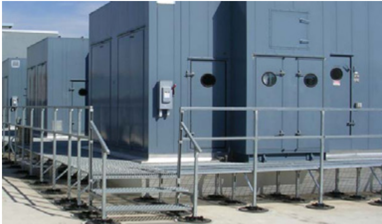
Access platform with stairs
