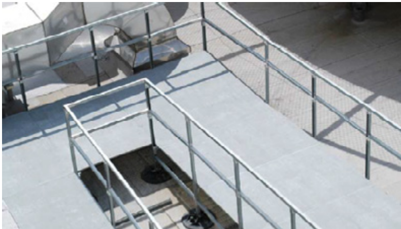
Ramp system with roof helipad access
