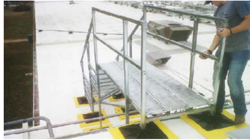
Roof-to-roof access stairs with handrails
