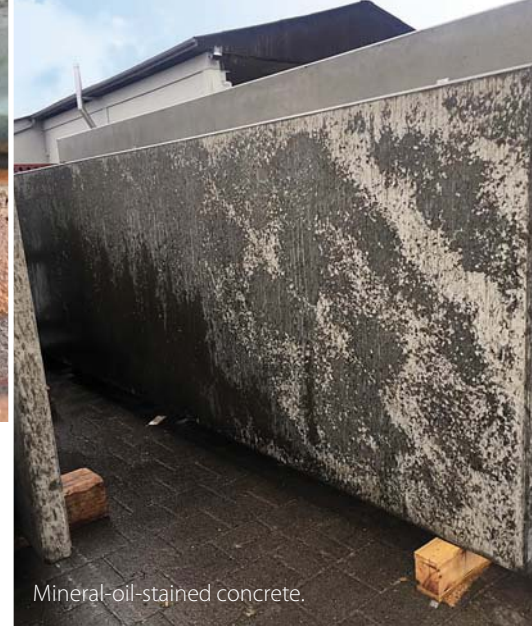
..... Friable concrete surface due to the over-application of oil.
