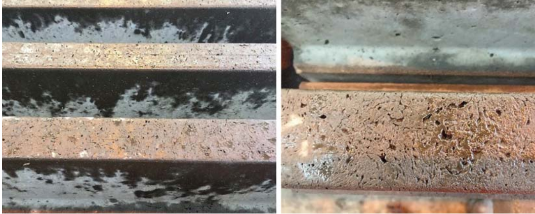
..... Friable concrete surface due to the over-application of oil.
