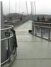
time, and move them over the bridge where they could be dropped into place. The low weight of FRP meant it was possible to place the panels from tower to tower and along the two back spans in around ten days.
