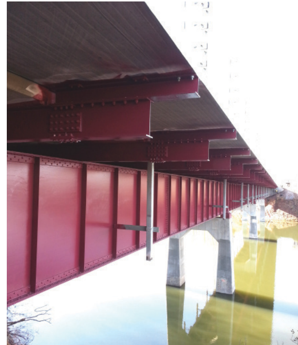
Recently-added cantilever footway on the Wilson-Burt Bridge in Niagara County, New York
