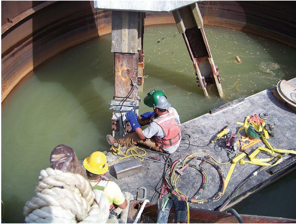
A crews installs the upper shear clips required for pier addition.
