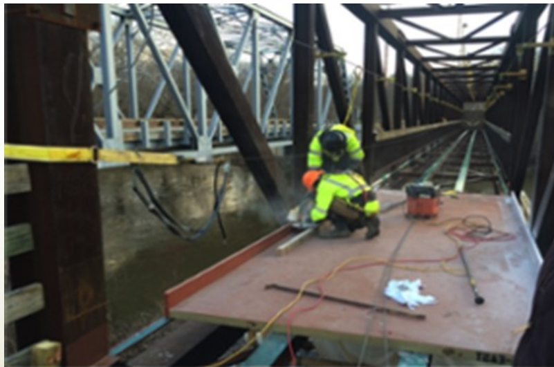
NPS installed a long lasting FRP deck after closing Cuyahoga Valley National Park's Hillside Pedestrian Bridge (right) in 2015 due to rotting timbers and corroding steel.
