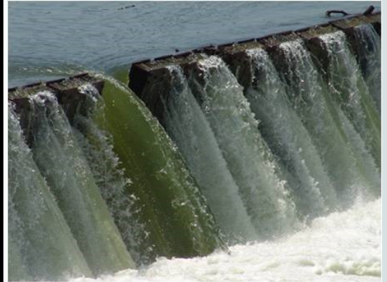
Wood wicket gates have short life spans and are not sustainable.
