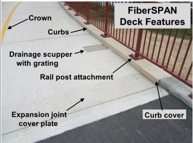
FiberSPAN panels weigh between 4 and 9 psf for a 80 percent weight savings when compared to concrete decking. Sidewalk components are prefabricated to reduce installation costs and speed construction. Features like those illustrated above can also be added during prefabrication. A sidewalk system featuring stringers, deck and railing can weigh as little as 16 psf.
