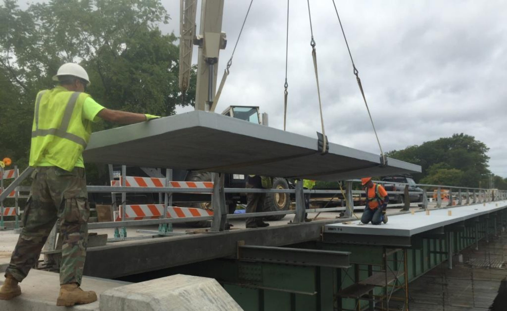
Final panel placement for Wilson-Burt Bridge cantilever sidewalk
