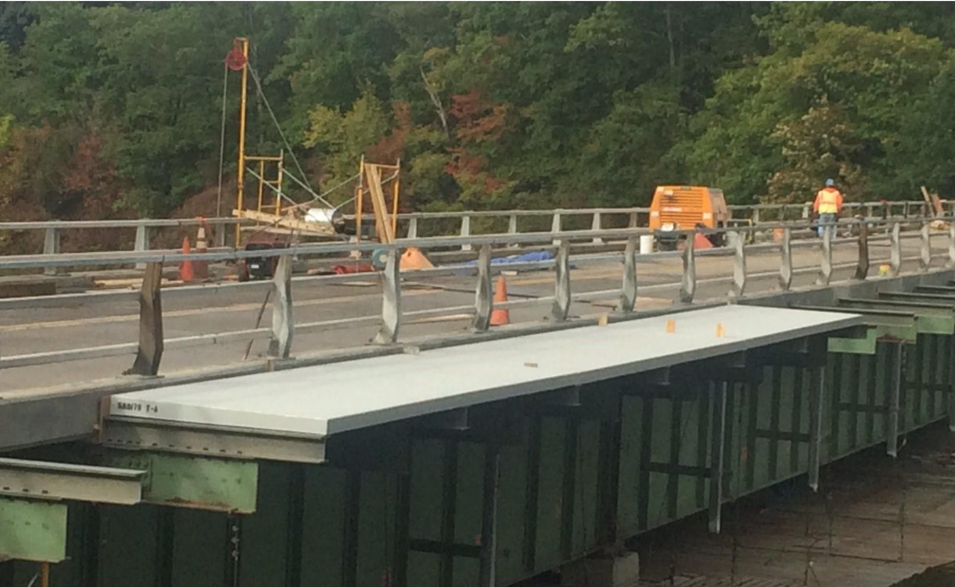
First panel installed on Wilson-Burt Bridge cantilever sidewalk
