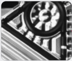
Fully drained leak detect
