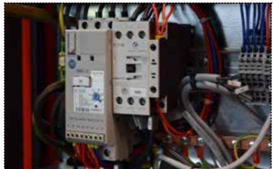
Motor **soft-starter** allows a reduction of the load and torque in the power train and electrical current surge of the motor during start-up. This reduces the mechanical stress on the motor and shaft, as well as the electrodynamic stresses on the attached power cables and electrical distribution network, extending the lifespan of the system.
