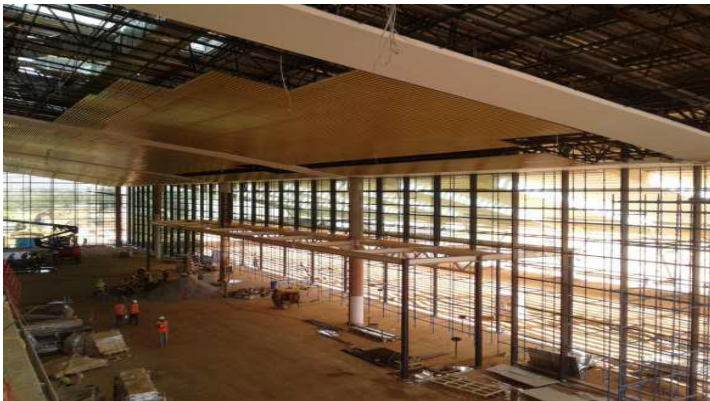
Figure 5: New terminal building, 23 February 2019
