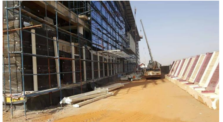
Figure 4: New terminal building, 23 February 2019
