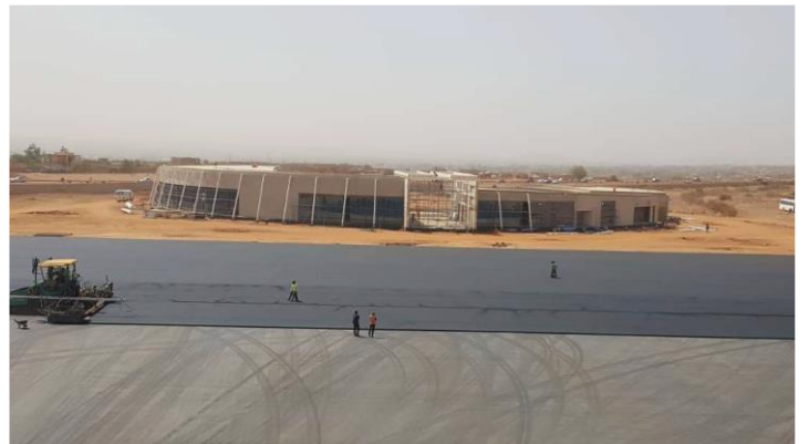
Figure 6: Presidential pavilion and apron, 23 February 2019
