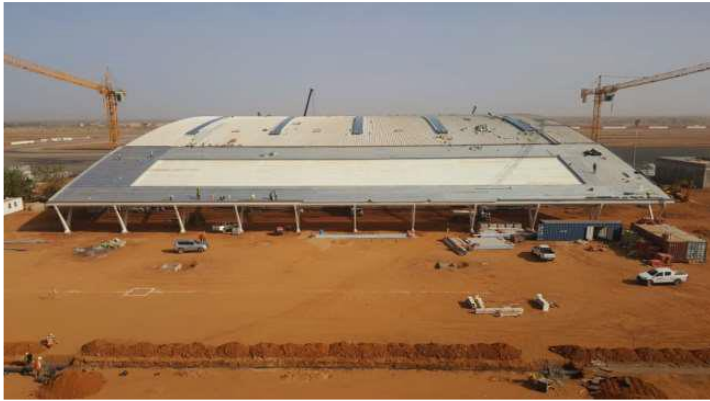
Figure 3: New terminal building, 23 February 2019
