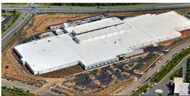
Subject Data Center
