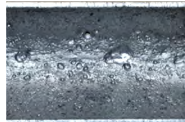
Under Deposit Oxygen Corrosion
