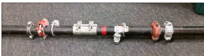
Multiple Leak Repairs on a Single Branch Line
