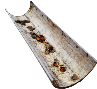
Corrosion assessments, pipe analysis, and long term corrosion control programs to mitigate future risk
