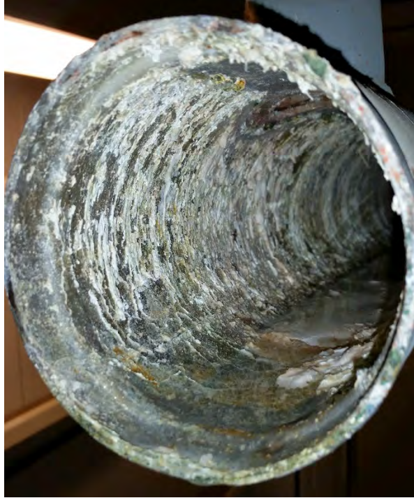
Figure 3: Freezer System Piping Maintained by Nitrogen Gas
