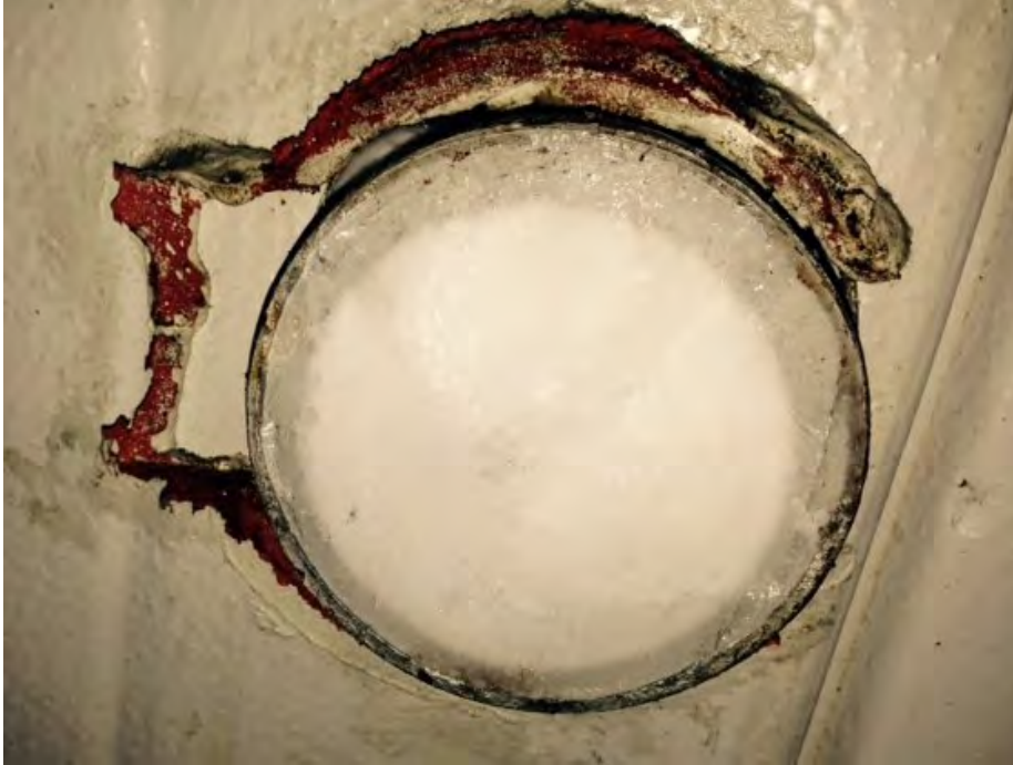
Figure 1: Ice Plug formed inside of Freezer System
