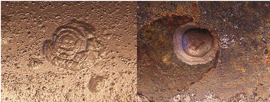
Figure 1: Microbiologically Influenced Corrosion (MIC) Pit (left) vs. Oxygen Corrosion Pit (right)
