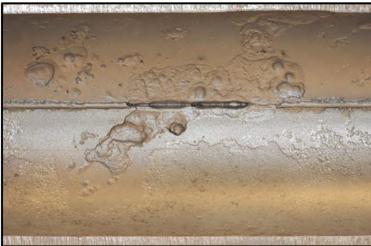
Figure 4. Weld Seam Corrosion of 4" Galvanized Main
