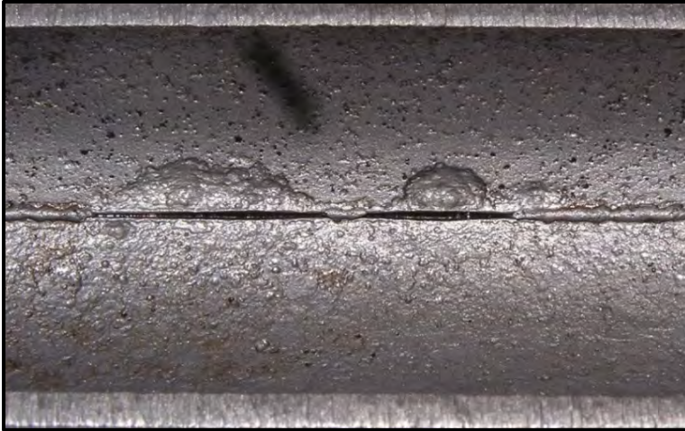
Figure 3. Knife-Cut Corrosion of 1" Black Steel Branch Line
