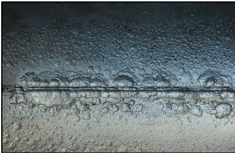
Figure 7. Severe Metal Loss in the HAZ resulting from Under-Deposit Corrosion (Vertical Riser Pipe)
