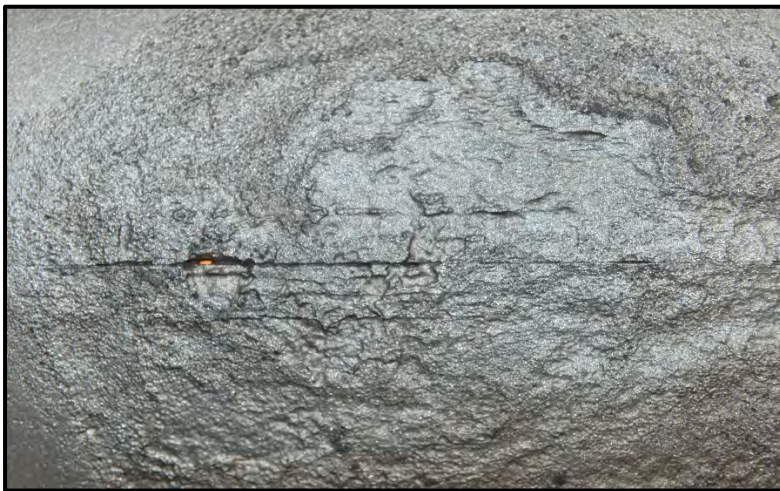
Figure 6. External Corrosion Resulting from Leak, with additional Metal Loss at Weld
