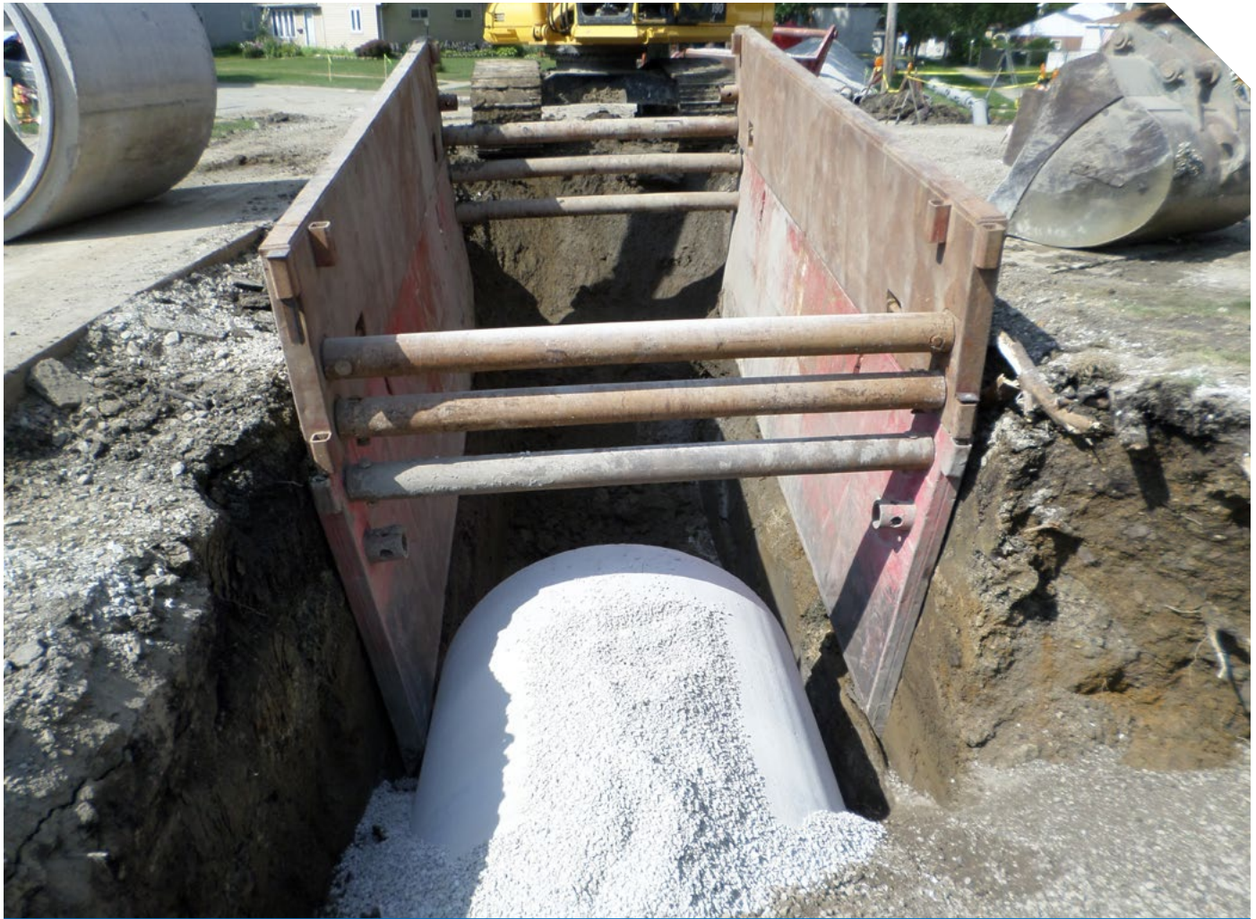
Installation of 84-inch combined sewer along Isabella Street.
