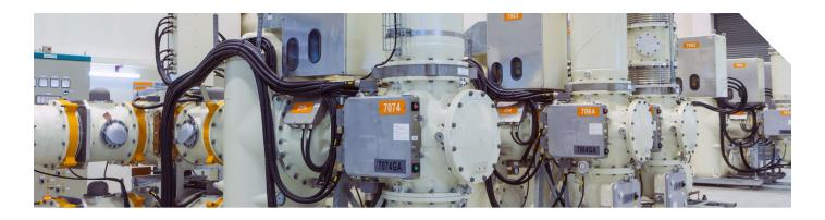
the underground system. The other four terminal positions are dedicated to four transformers. The low side of each transformer remained as it was connected prior to the retrofit, serving the existing 13.8-kV yard. Relaying and control systems use IEC 61850 for most operations, including fully separated primary and backup systems located within a new control enclosure.
