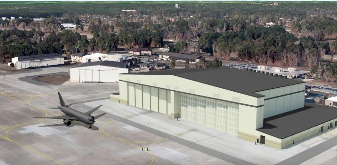
89,825 square feet of attached shops. Shop areas include spaces for administrarative offices, bathrooms, locker rooms, storage, aerospace ground equipment, hydraulics and brakes, corrosion control, fuel cells, and nondestructive inspections.
