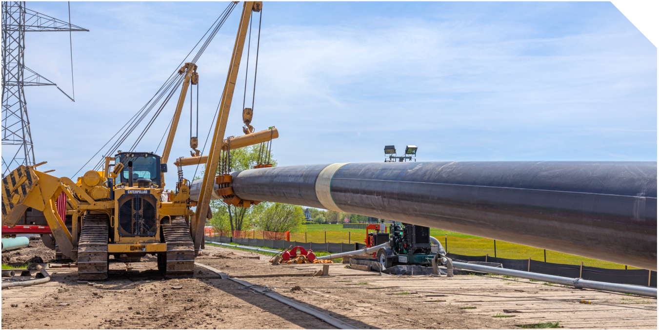
Installation of a natural gas pipeline.
