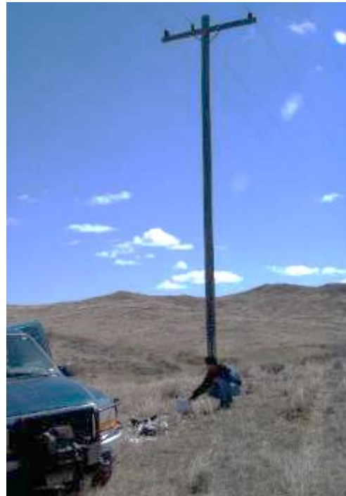
3-phase on flat top design with no neutral
