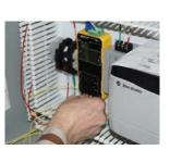
through the equipment and attach to the HSM module inside the low voltage compartment.
