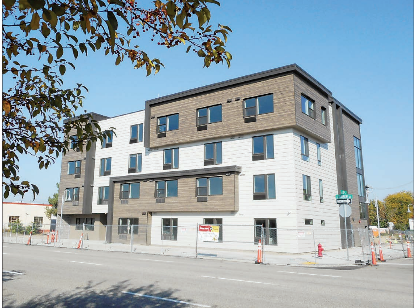
The New Path Community Housing project during last year's construction.
