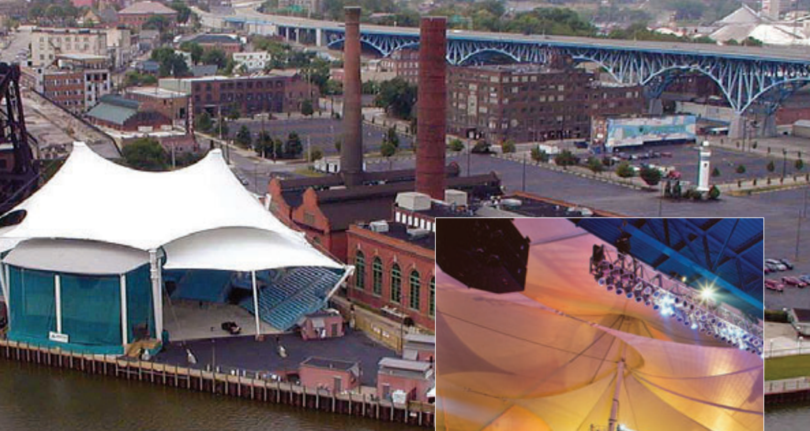
The pavilion design was inspired by the free forms of surrounding rivers and bridges.
